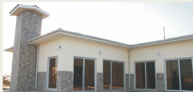
Wall Tile and Cement Board
