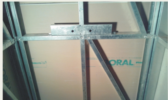
Wash Basin Fixing Arrangement
