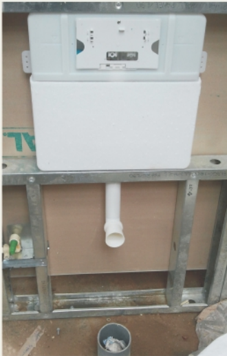
Wall / Floor mount WC Fixing Arrangement
