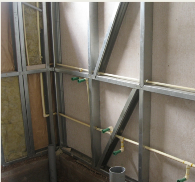
Arrangement of Pipe line for Various Services
