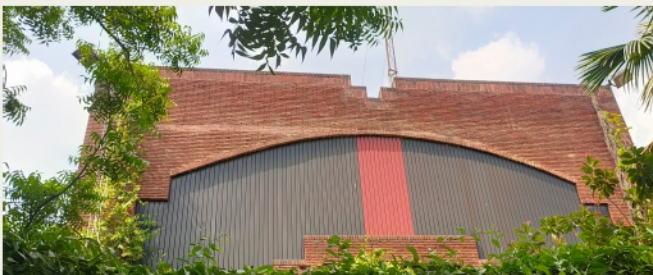
Exposed Brick Cladding
